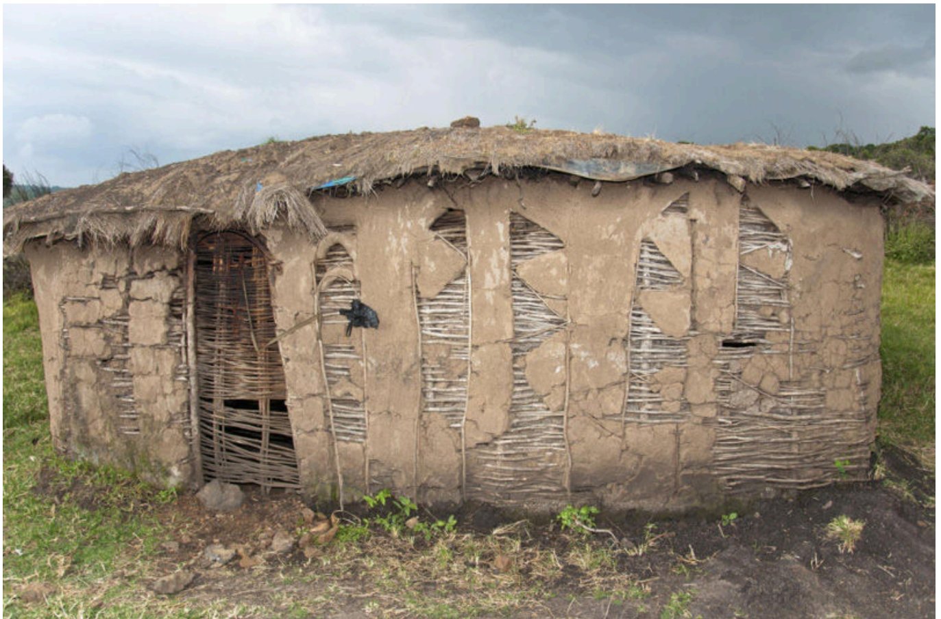
Wattle and daub construction technique
