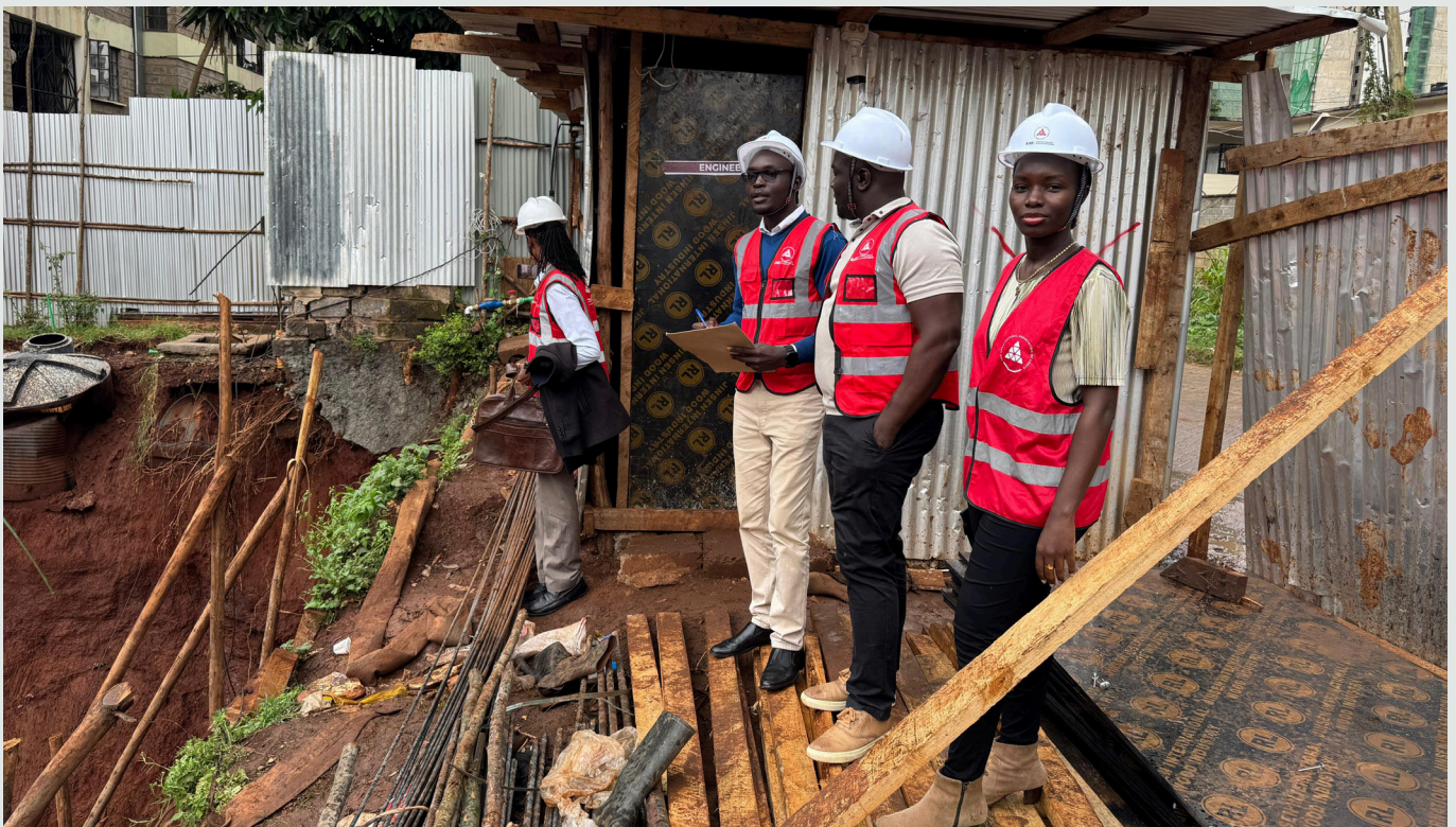
Mulika Mjengo site inspection at Suswa Road, Parklands
