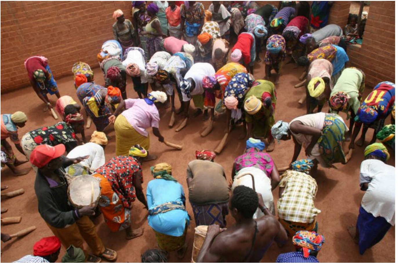
Community members flattening the floor during the construction of the Gando Primary School Extension. Source: Kéré Architecture.
